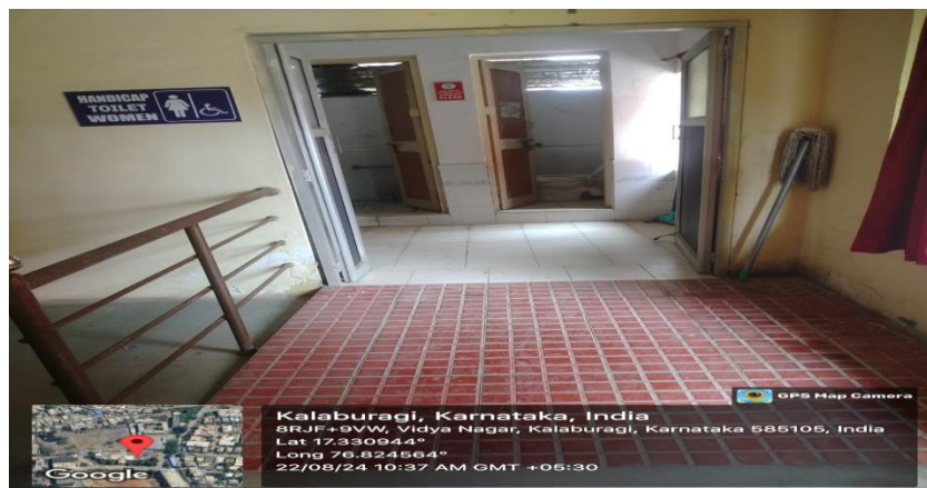
SUK BLOCK 5 PHYSICAL HANDICAP TOILET
